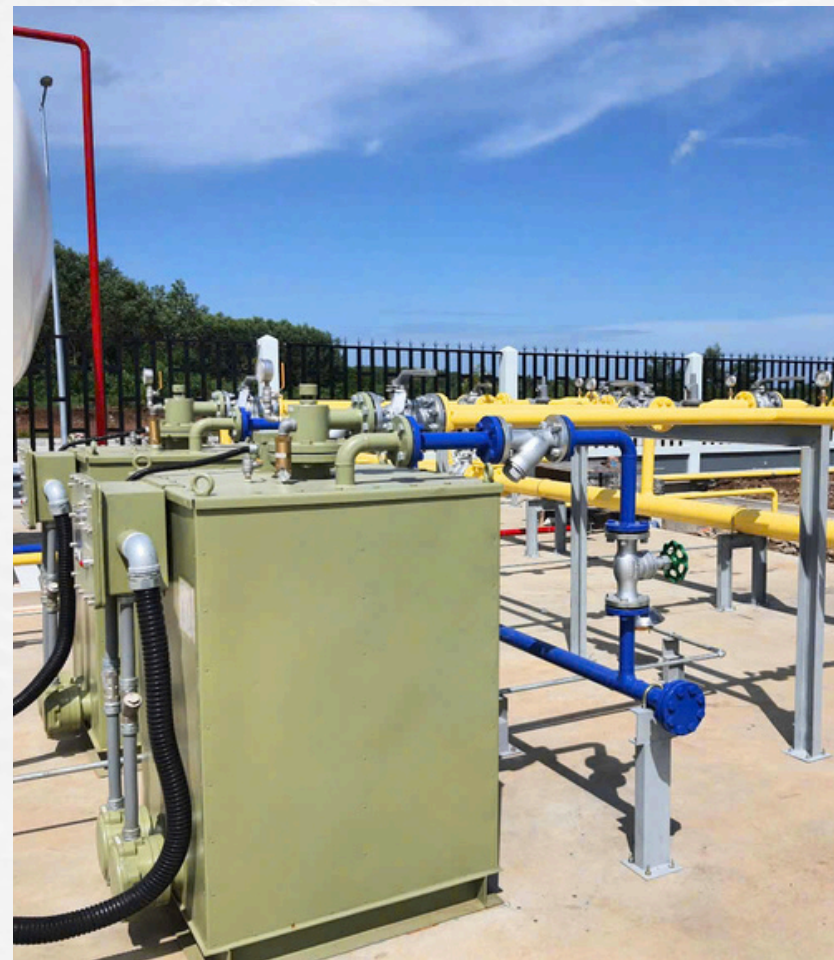
Electric vaporizer at site and MSEng Viet Nam's Valve
