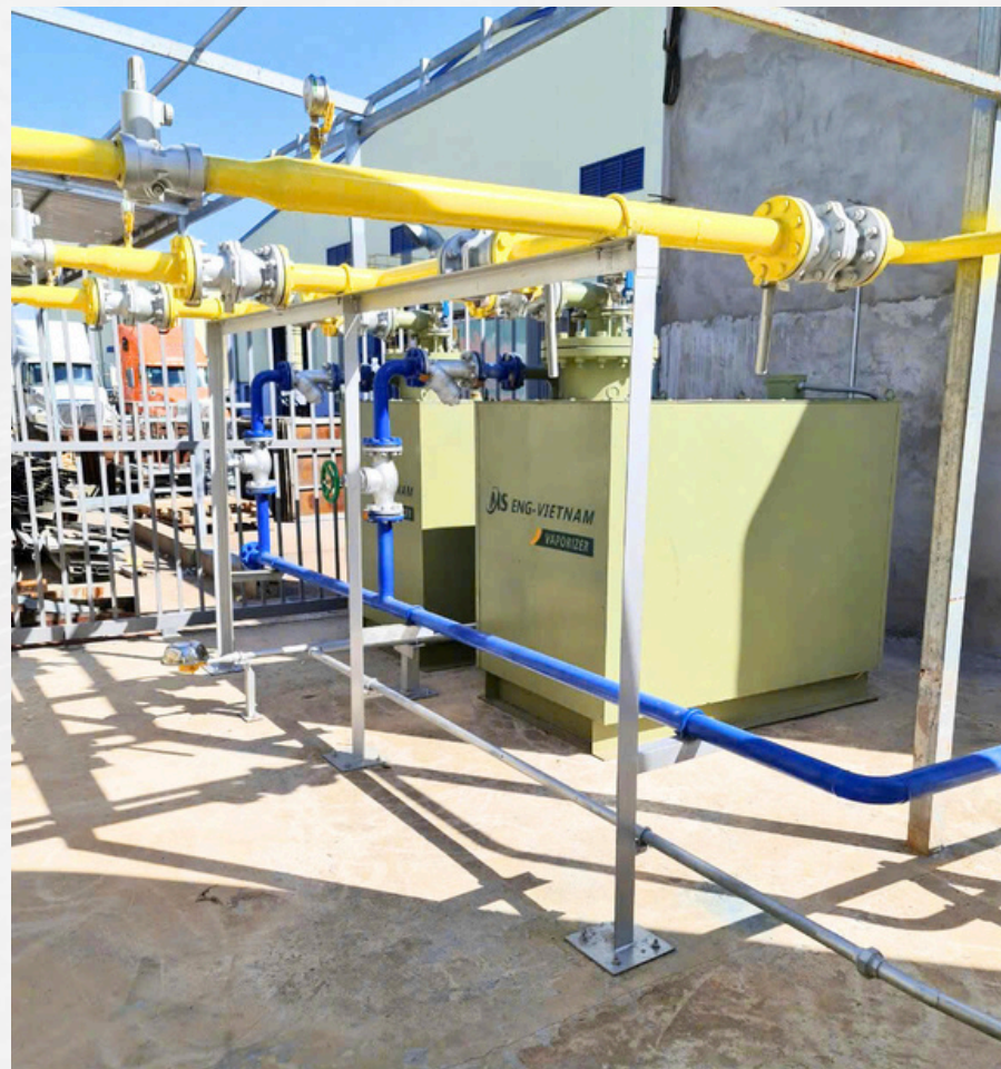
Electric vaporizer at site and MSEng Viet Nam's Valve
